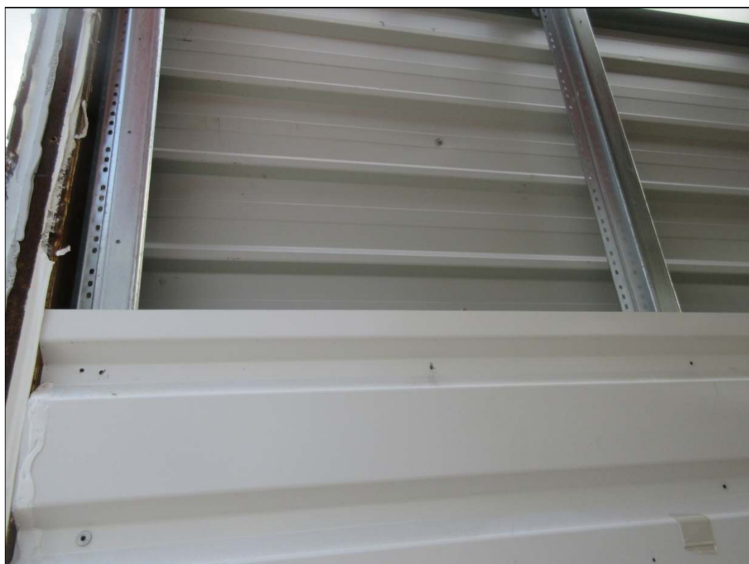
SAMPLE DURING DISMANTLE
