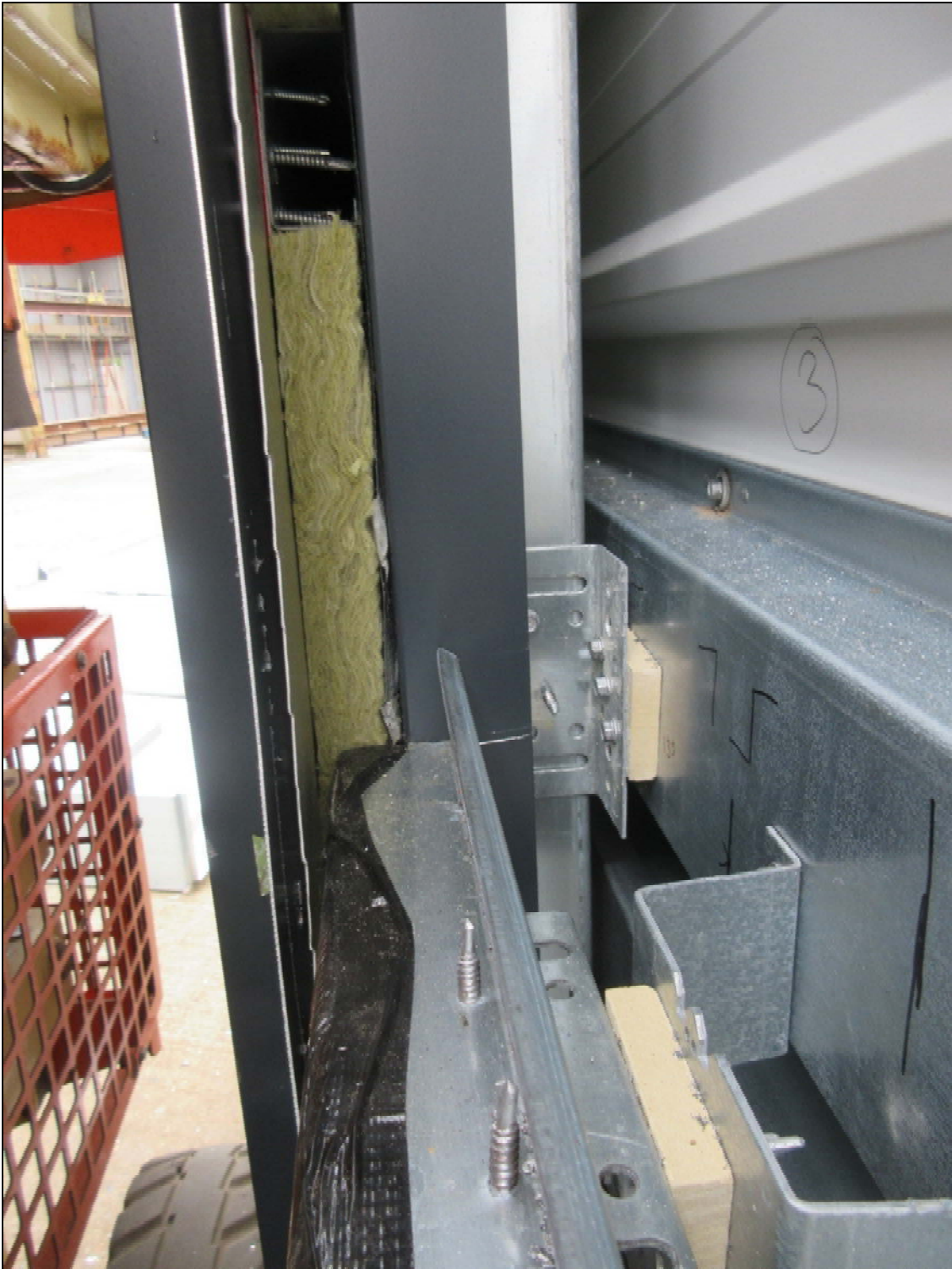
SAMPLE DURING DISMANTLE
