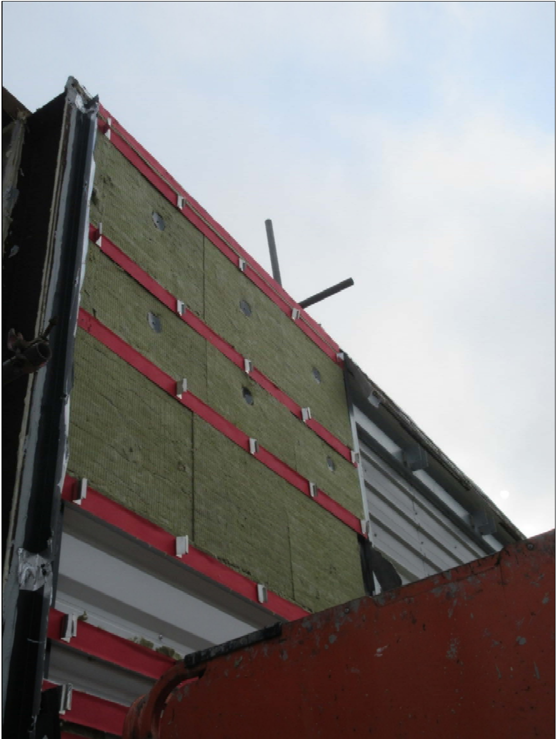
SAMPLE DURING DISMANTLE
